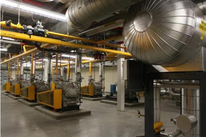
The refrigeration plant also boasts a redundancy factor and design provisions that would allow the Enerplex to tie into, and refrigerate, the neighboring ice facilities if needed in the future. Additionally, the Enerplex has the ability to capture 75 percent of its waste heat which is used to heat the domestic hot water, spectator areas, and the snow melt pits.
