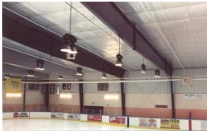
Figure #3 - Typical EnerShield Low Emissivity Ceiling Installation
